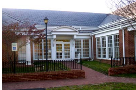
The expanded Cochrane-Rockville Branch Library opened to the public in October 2005.
